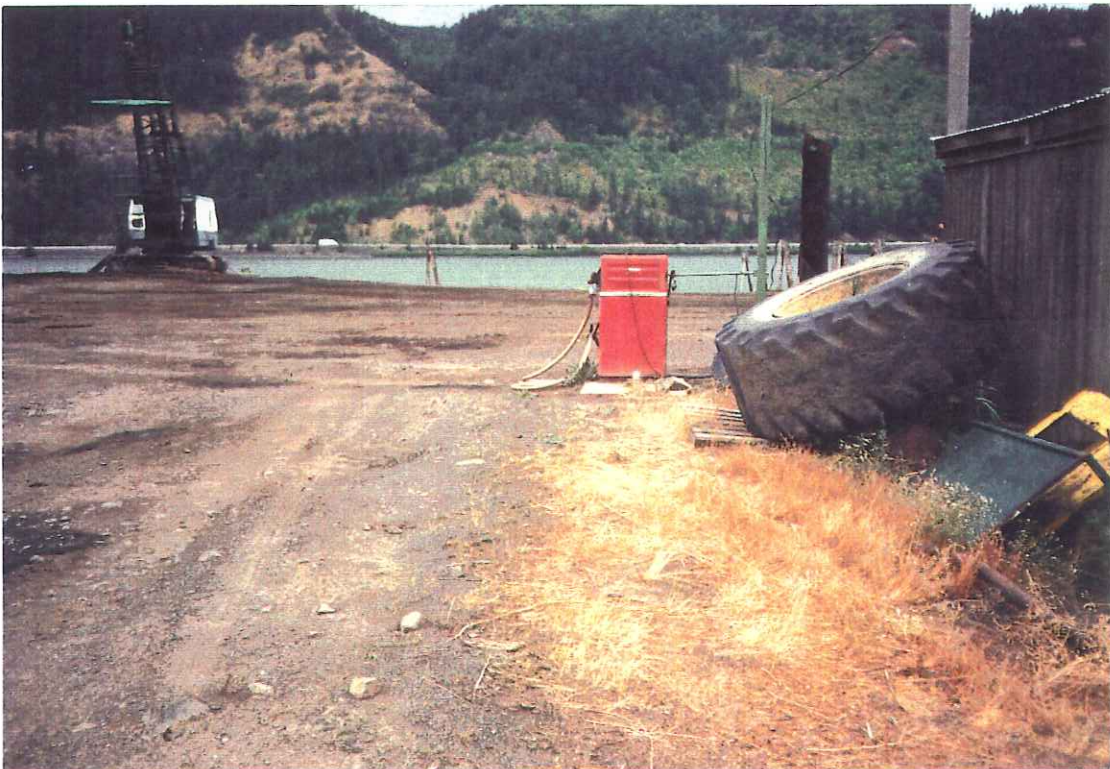
Pump above Underground Storage Tank in Log Yard
