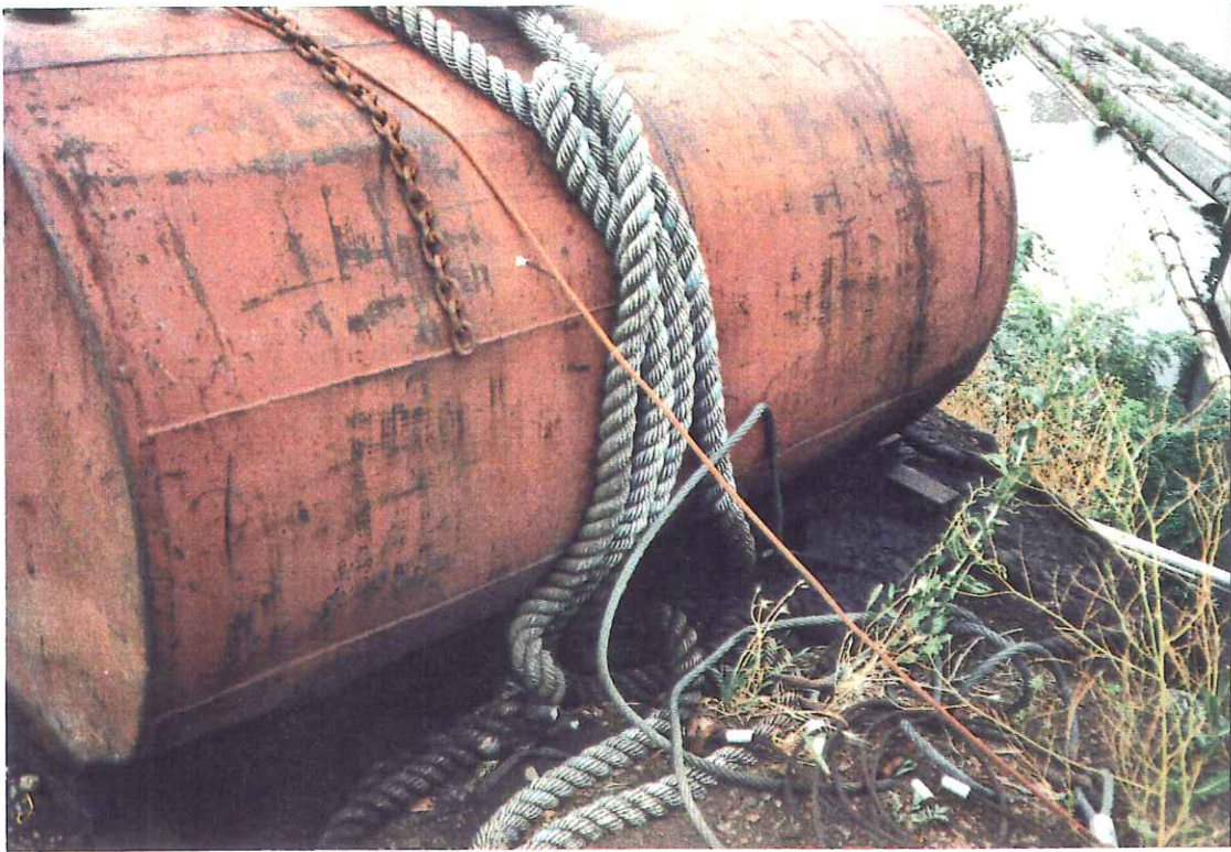
Above Ground Storage Tank in Log Yard Area
