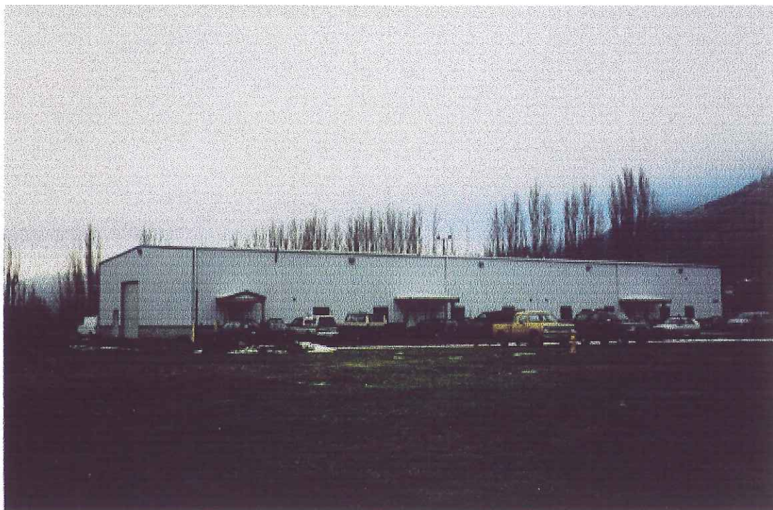
4.5 Typical Light Industrial Park Building: Small Business Development Center at Bingen.
